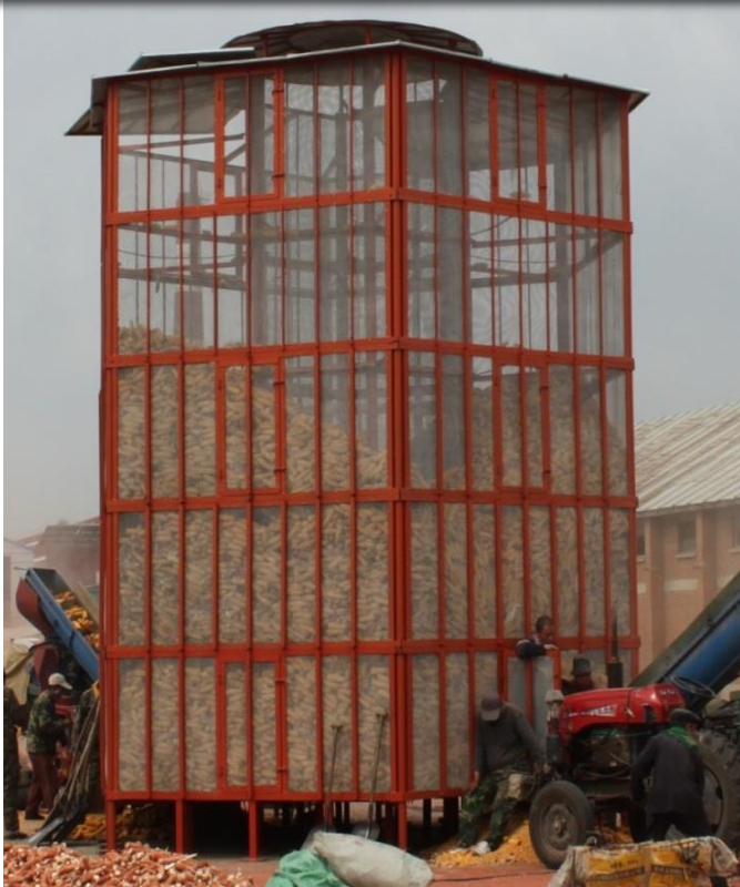
钢骨架六角环形仓 Hexagonal ring silo with steel skeleton
