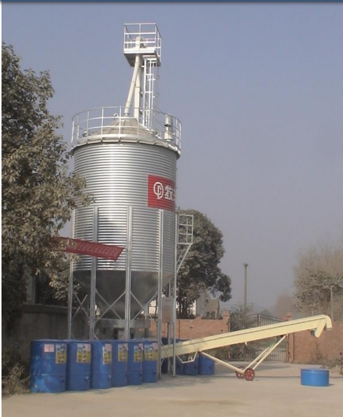
农户小型钢板仓 Small steel silos for farmers
