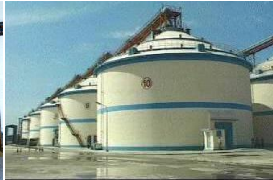
concrete squat silo
