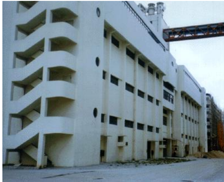
multi-storied warehouse reinforced
