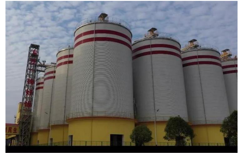
silos 隔热钢板仓
