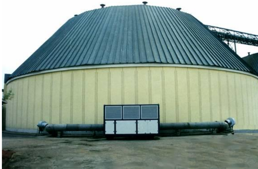
Grain cooler for squat silo 浅圆仓谷冷机
