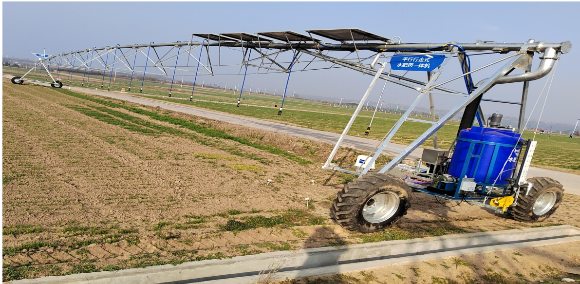
Line-moving springkler irrigation with solar-powered
